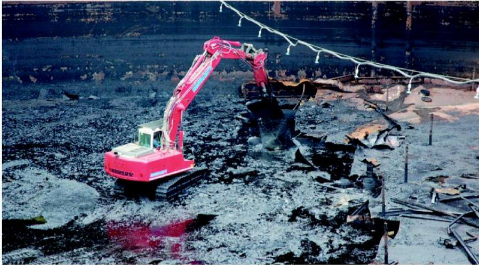
unbalanced. Once the support legs reached the bottom, they crippled under the excessive weight. As the roof collapsed from the pressure below, it had practically come to rest on the floor of the tank.
